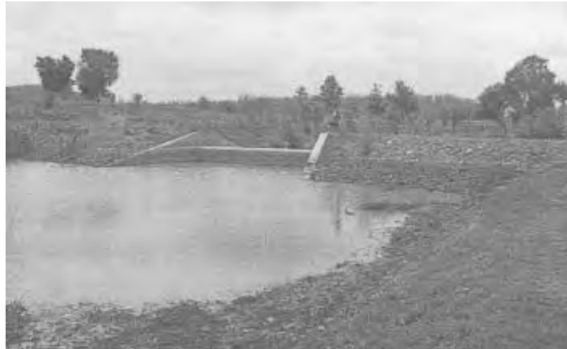
A small dam
