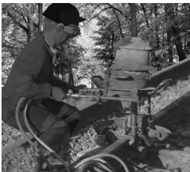
Figure 3.11 Thermit process for joining railway tracks
